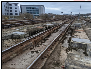
Fig 5.7 Old Train Wash Foundations
